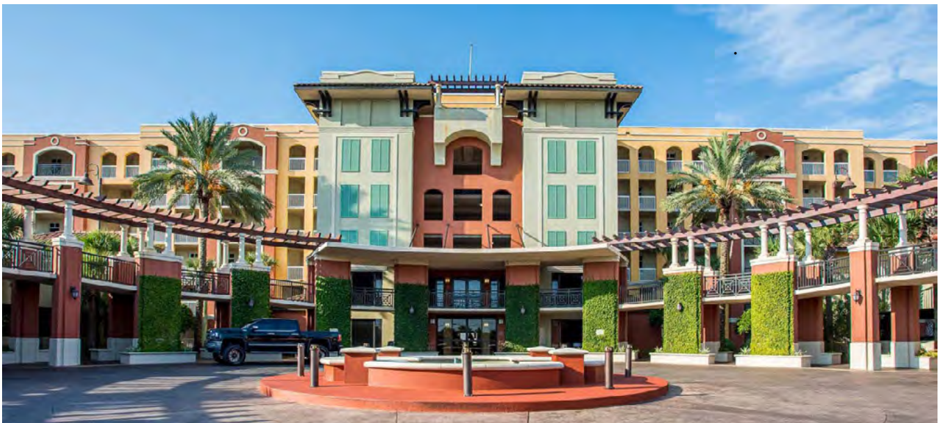
Image: Azure - 2024 Exterior Restoration Design Project
