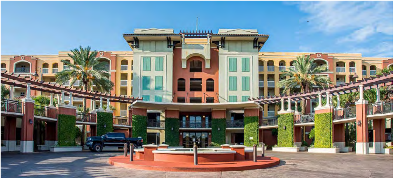
Image: Azure - 2024 Exterior Restoration Design Project
