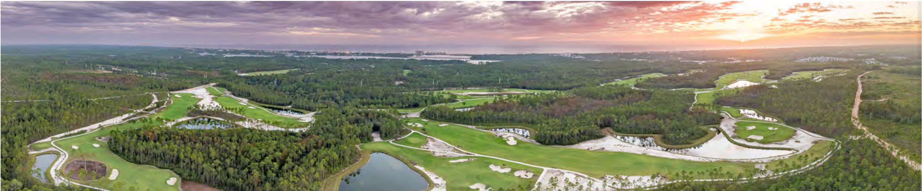
Image: 3rd Golf Course ~ 2023 Civil Engineering Project
