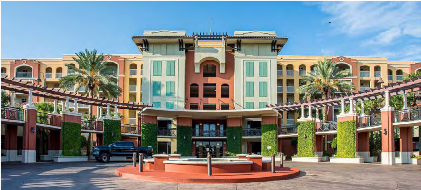
Image: Azure - 2024 Exterior Restoration Design Project
