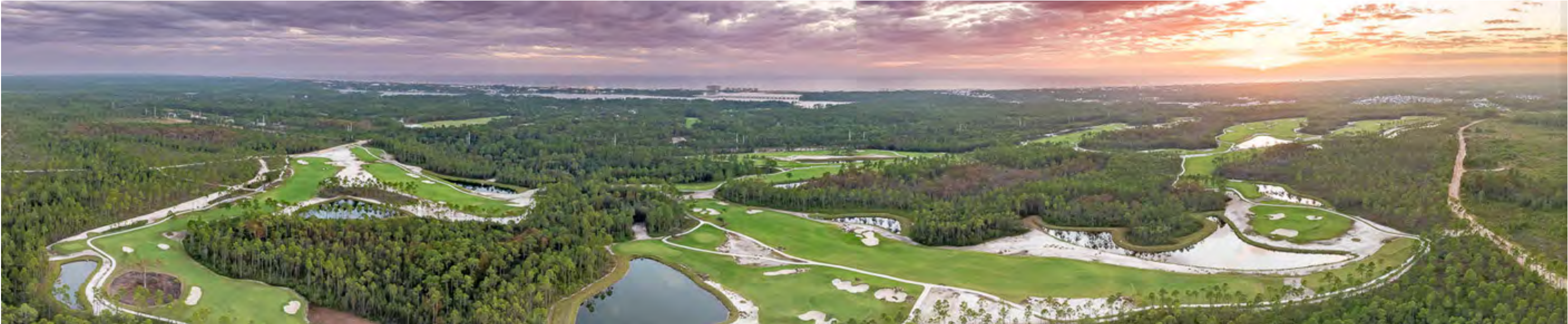
Image: 3rd Golf Course ~ 2023 Civil Engineering Project
